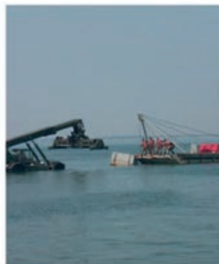
Recovery Operation using the RTCH
